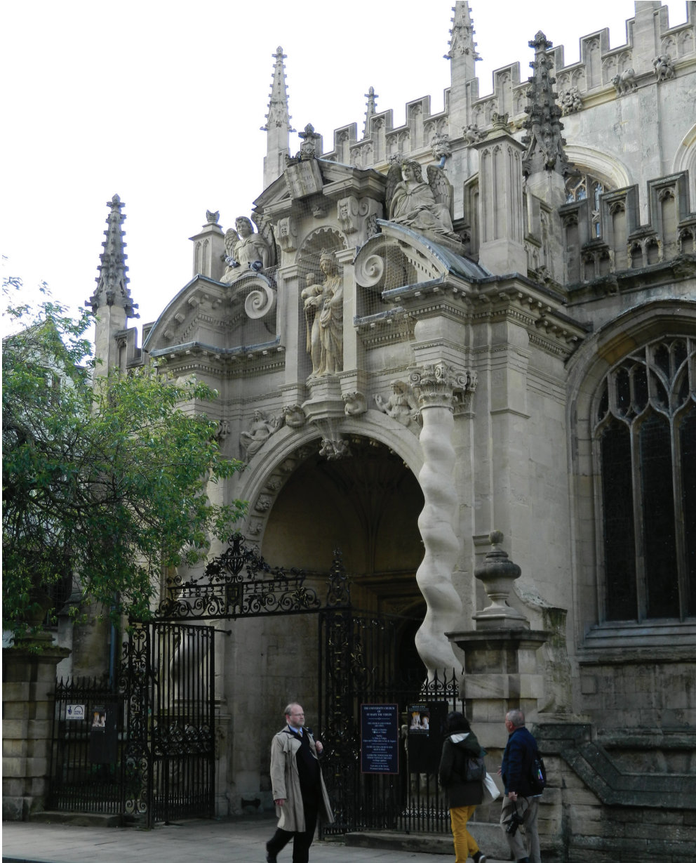
Fig. 4. South porch of St Mary's, by John Jackson, 1637. Height approximately 8 metres. Photo: Robin Usher.
